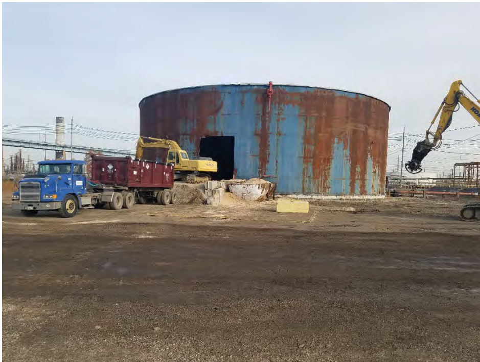
Photograph 2: View of Tank 016A (GP R 227) during demolition.
