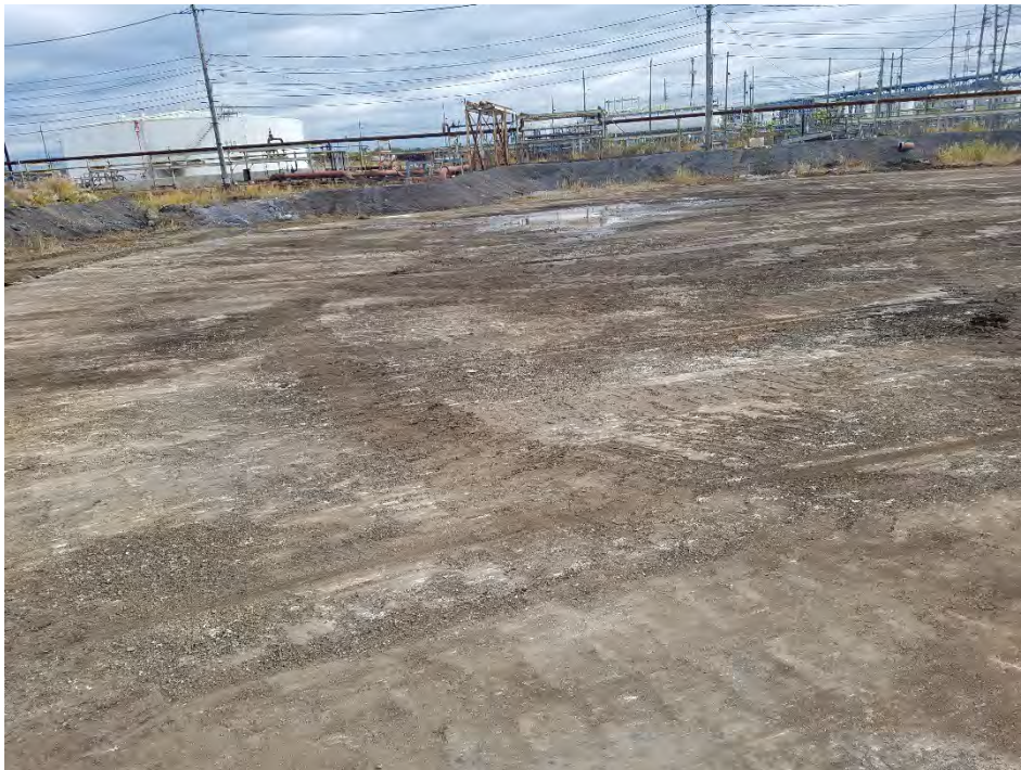
Photograph 2: View of Tank 015A (GP R 225) concrete pad.
