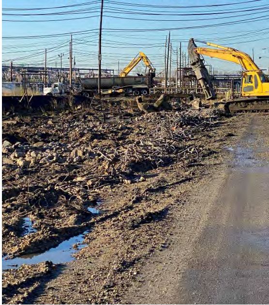
Completed loadout at GP219
