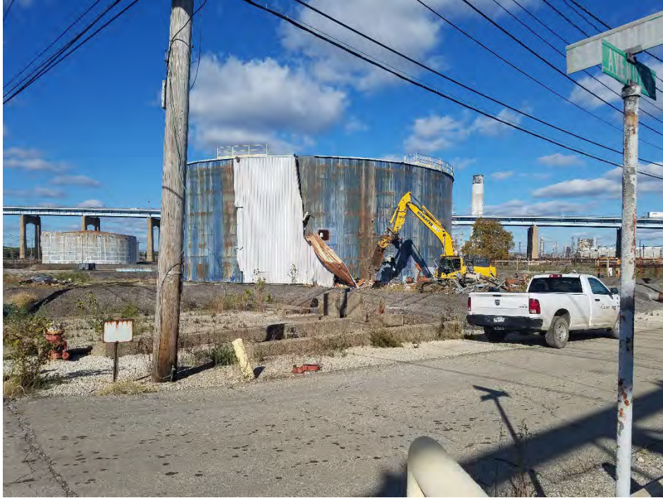
Photograph 1: View of Tank 015A (GP R 225) during demolition.
