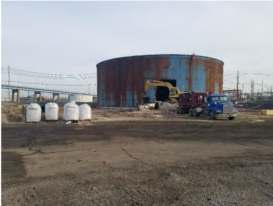
Photograph 1: View of Tank 016A (GP R 227) during demolition.
